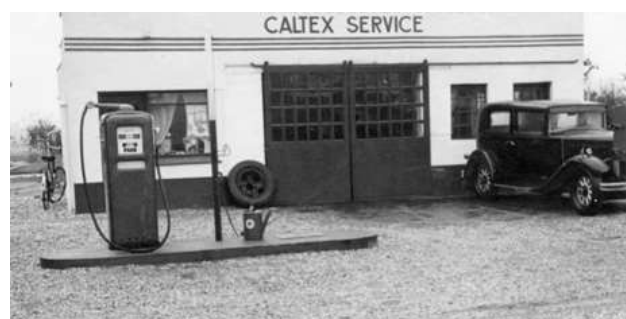
Servicestationen Vestergade 42 i Auning.
